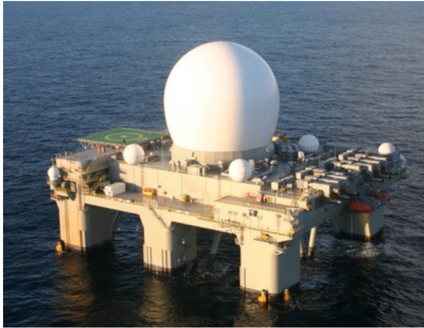
SBX ballasted down in stable “semi-submerged” operating position
