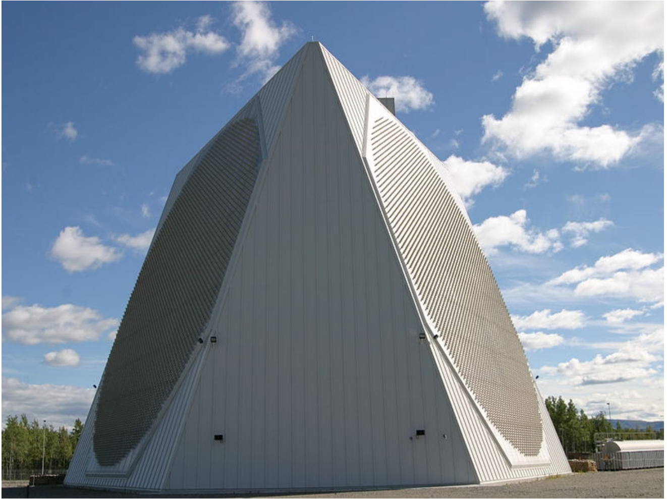
Ground-level view of two-antenna Pave Paws installation at Clear AFB, Alaska
