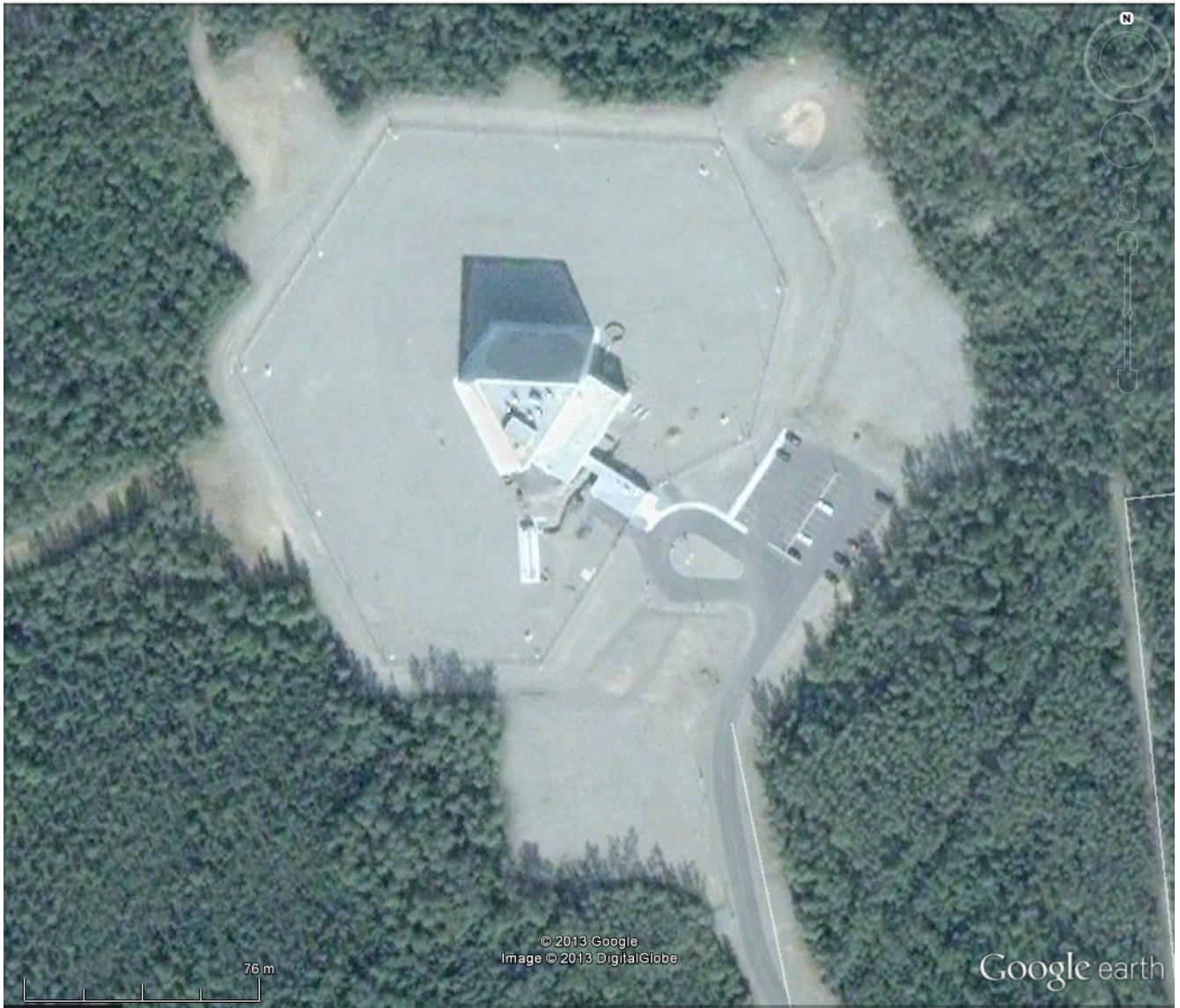
Overhead view of two-antenna Pave Paws installation at Clear AFB, Alaska
