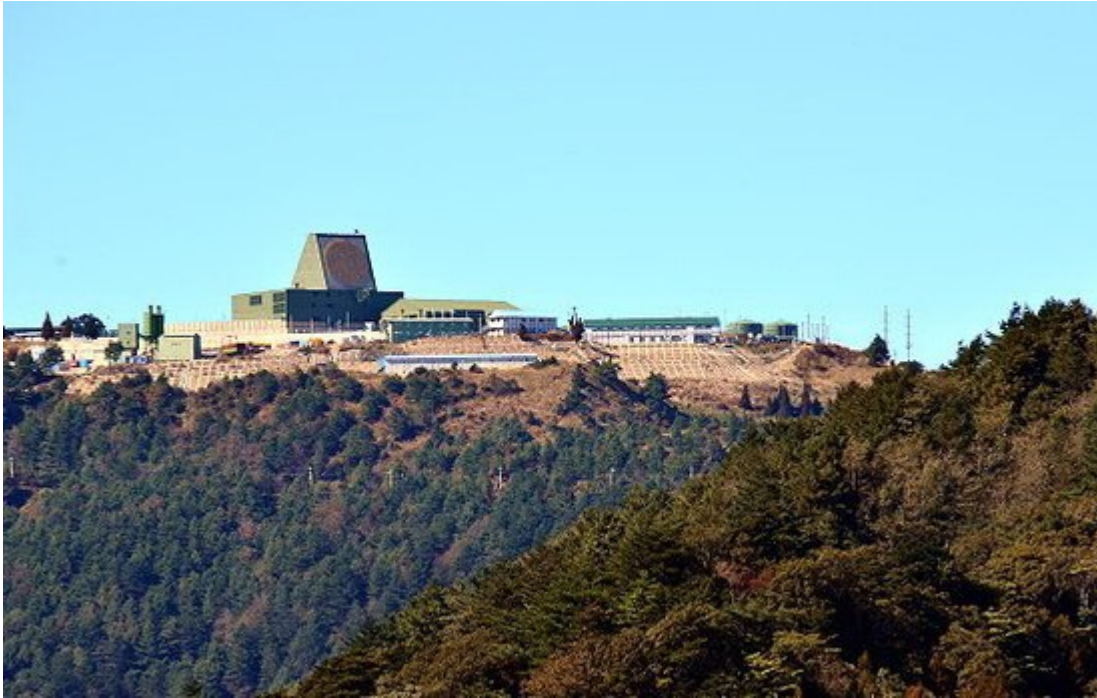
Data Figure: Taiwan's Hsinchu Leshan base PAVE PAWS radar facilities
