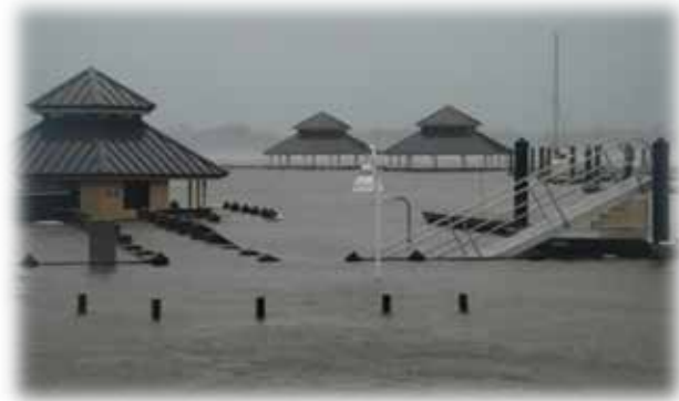
Flooding at Keesler Air Force Base. Credit: SSgt Kimberly Rae
