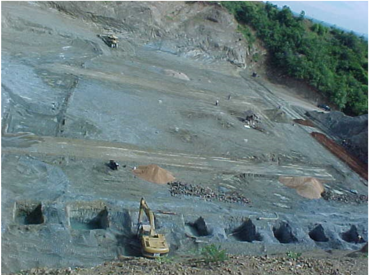
preparing the concrete pad and support beam holes
