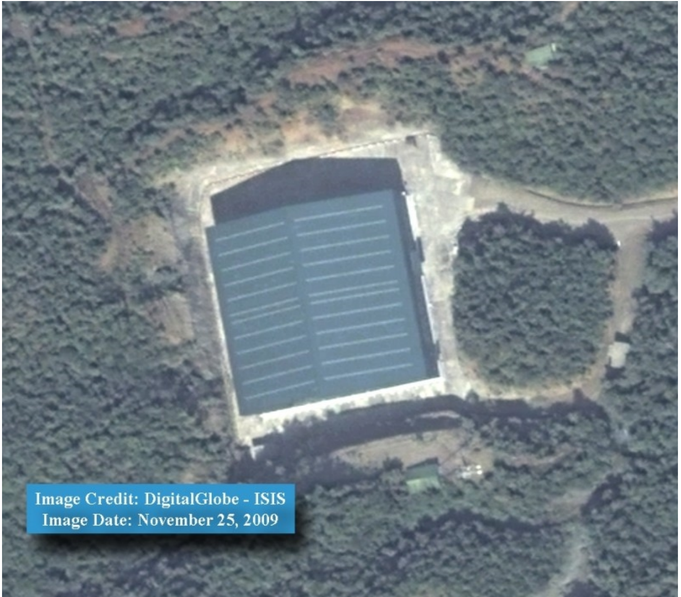
Figure 3. ISIS learned that another set of the high precision equipment in the first building was also sent to this building.
