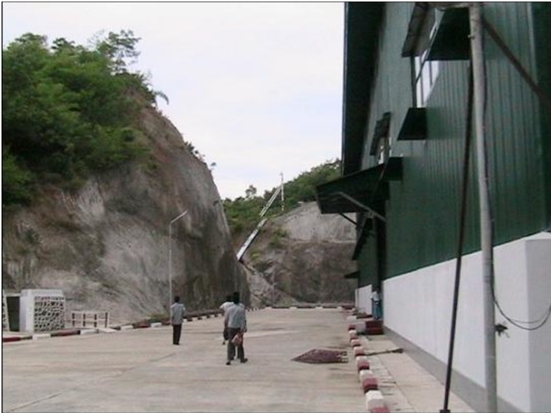
stabilizing the surrounding banks with shotcrete
