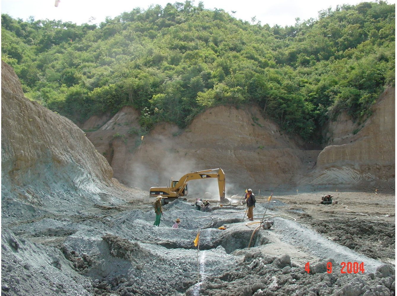
clearing the forest and leveling the ground
