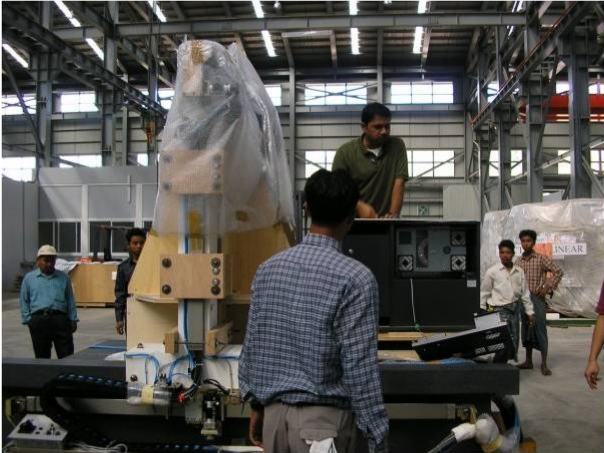
installing the CNC machines
